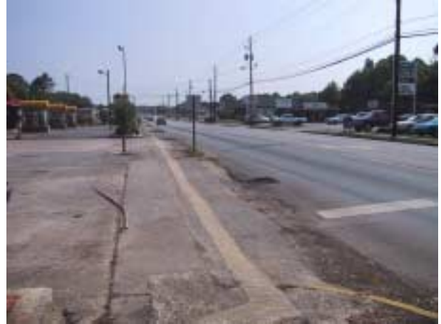
Excessive Number of Driveways – North Main Street at East Girard Avenue
